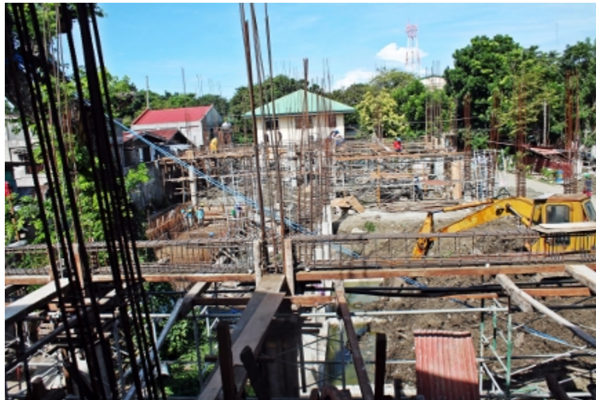
The construction of new buildings. Source: WVCST.
